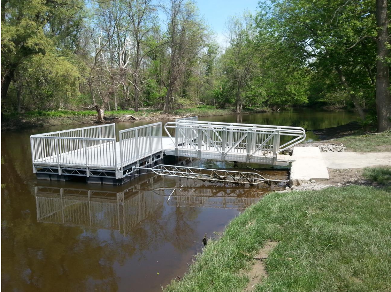
Dock on Black Creek
